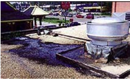
Roof Without Grease Guard Protection Roof Without Grease Guard Protection
