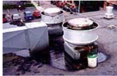
Roof Without Grease Guard Protection Roof Without Grease Guard Protection
