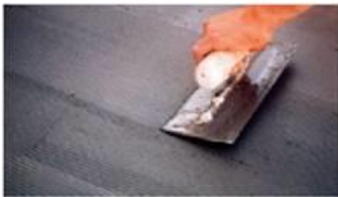
Apply Bonding Agent (latex modified thin-set).
