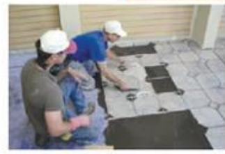
Install Tile by a Thin-Bed Method.
