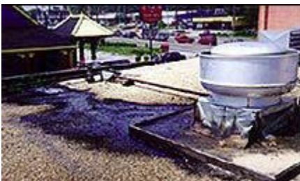
Roof Without Grease Guard Protection
