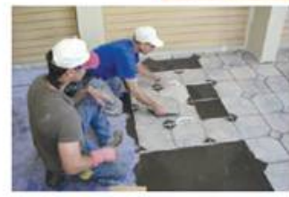
Install Tile by a Thin-Bed Method.
