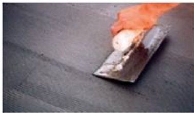
Apply Bonding Agent (latex modified thin-set).
