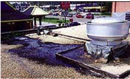
Roof Without Grease Guard Protection
