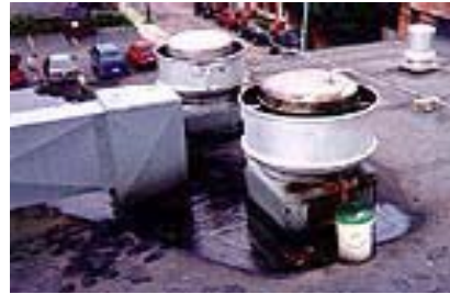
Roof Without Grease Guard Protection
