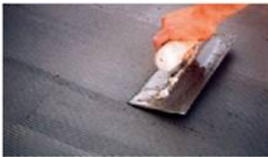
Apply Bonding Agent (latex modified thin-set).
