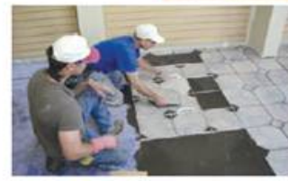
Install Tile by a Thin-Bed Method.
