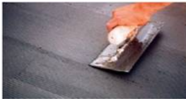
Apply Bonding Agent (latex modified thin-set).
