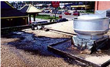
Roof Without Grease Guard Protection
