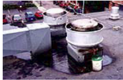
Roof Without Grease Guard Protection
