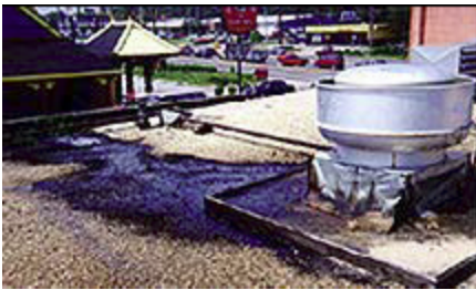
Roof Without Grease Guard Protection
