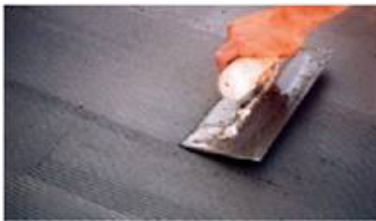
Apply Bonding Agent (latex modified thin-set).
