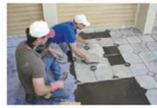
Install Tile by a Thin-Bed Method.
