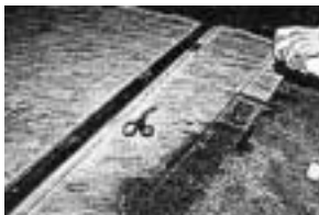
NobleSeal TS fabric coating must be removed to make a solvent weld where bare CPE seaming area is not provided. Flood areas to be seamed with Xylene approximately 1" wider than the seam marks.
