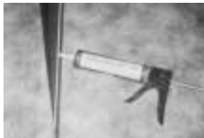
Apply first bead of NobleSealant 150 as shown.
