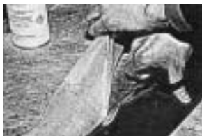
Cut fabric at the mark with scissors.
