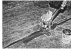
Use rubber roller to press seam together - removing air and excess solvent.
