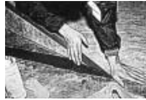
Press seam together while CPE is soft and wet.
