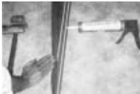
Apply second bead, then press seam.
