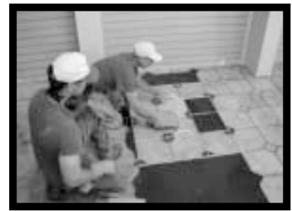
Install tile by a thin-bed method
