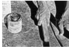
Roughen bonding area with copper scrub pad or clean wire brush to improve seam cement reaction.
