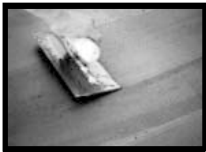
Apply bonding agent (latex modified thin-set)
