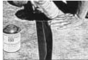
Position sheets side by side and overlap area to be welded. Prime/clean bonding area by lightly applying Xylene or alcohol.
